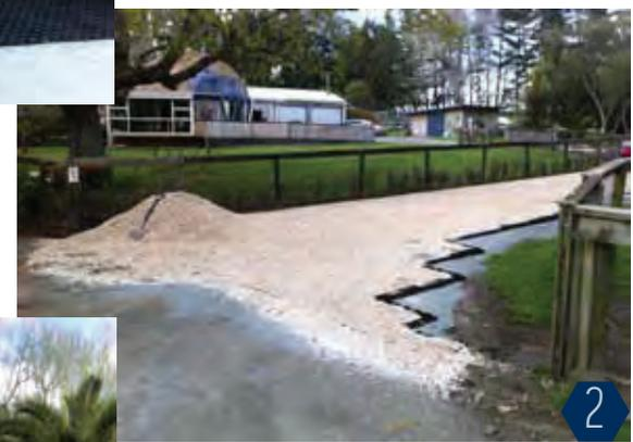
**JakMatGeocell** contains the materials in place, for heavy duty vehicles such as water trucks.
